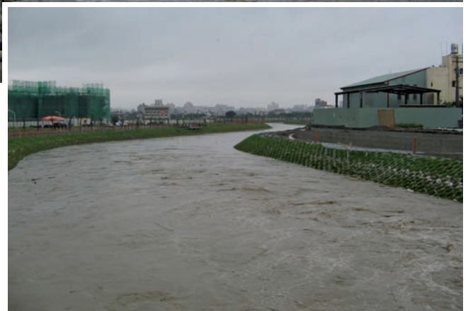
Finished channel at high water level just after the Morakot Typhoon hit Taiwan
