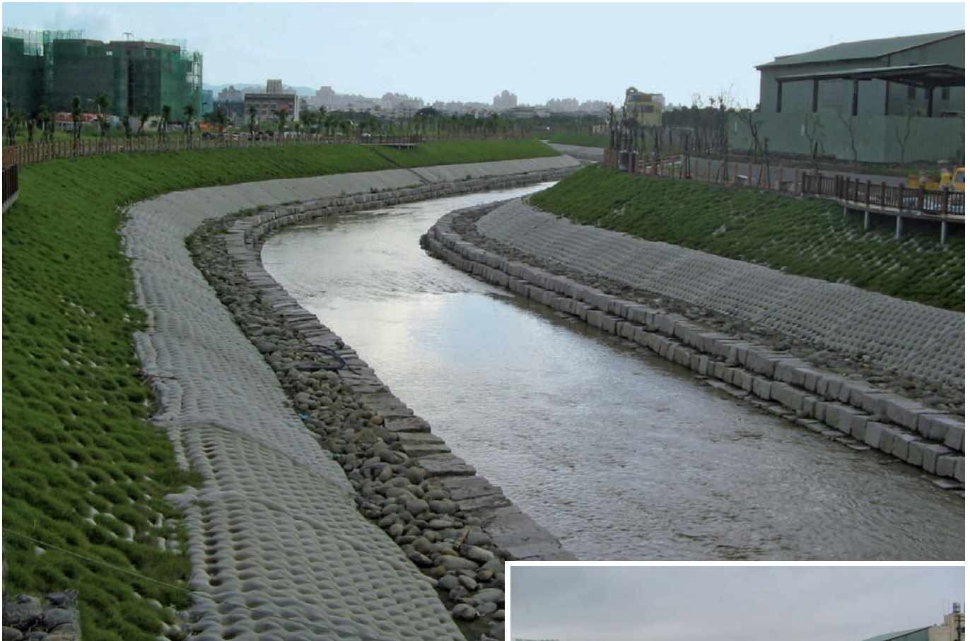
Finished channel shortly after completion
