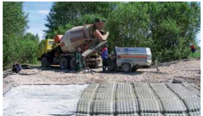
Installation of Incomat ® Flex
