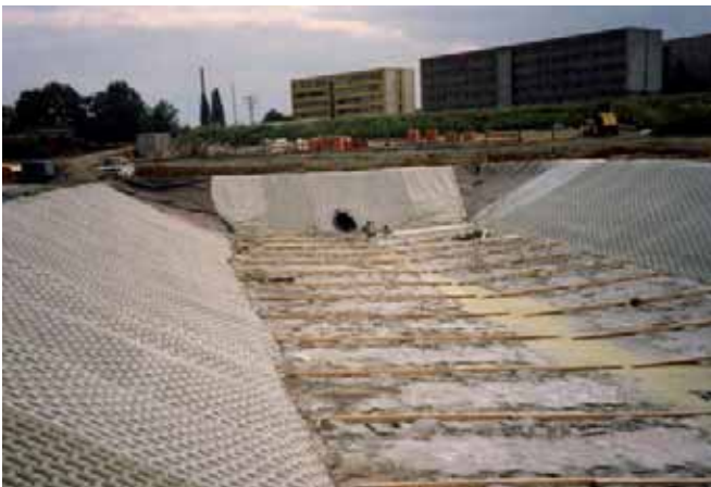
Attenuation pond with Incomat® Crib during construction (1)
