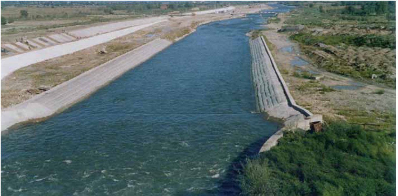
Slope protection with Incomat® Flex
