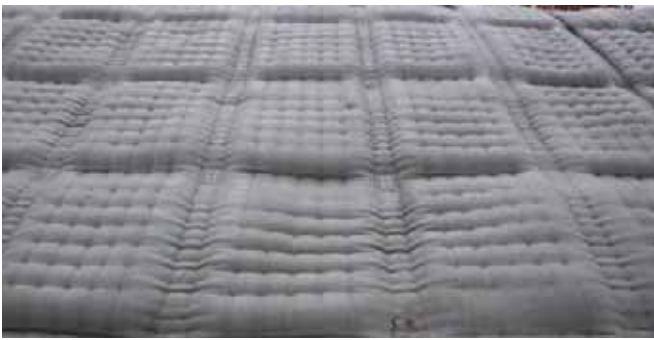
Incomat® Flex cushion mat for erosion protection with “hinged” intermediate junctions allowing certain flexibility and minor drainage through the mat by the incorporated drainage points.
