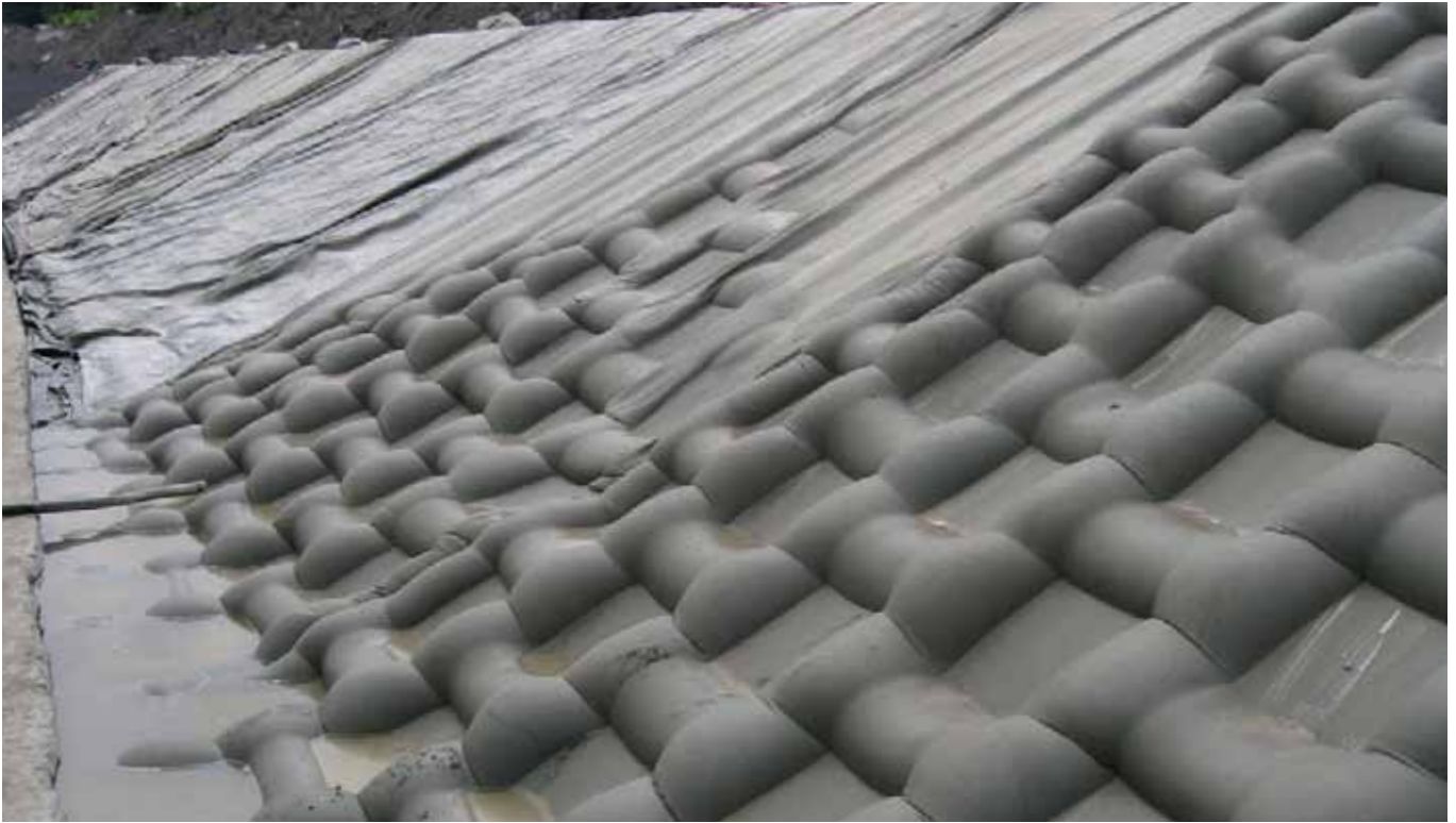
Installation of Incomat ® Crib
