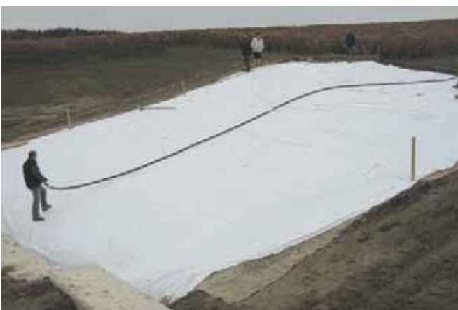
Incomat® FP prepared for installation (1)
