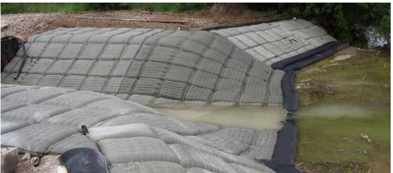
Repaired outlet after completion (4)
