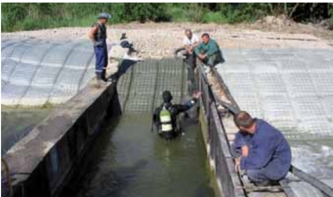
Installation of Incomat ® Flex under water
