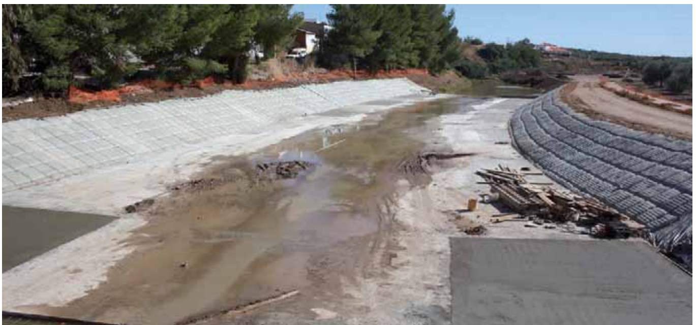
Slope protection with Incomat® Flex
