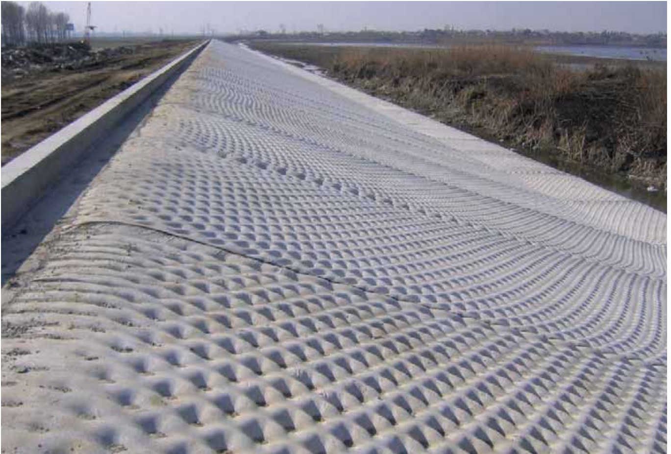
Slope protection with Incomat® FP
