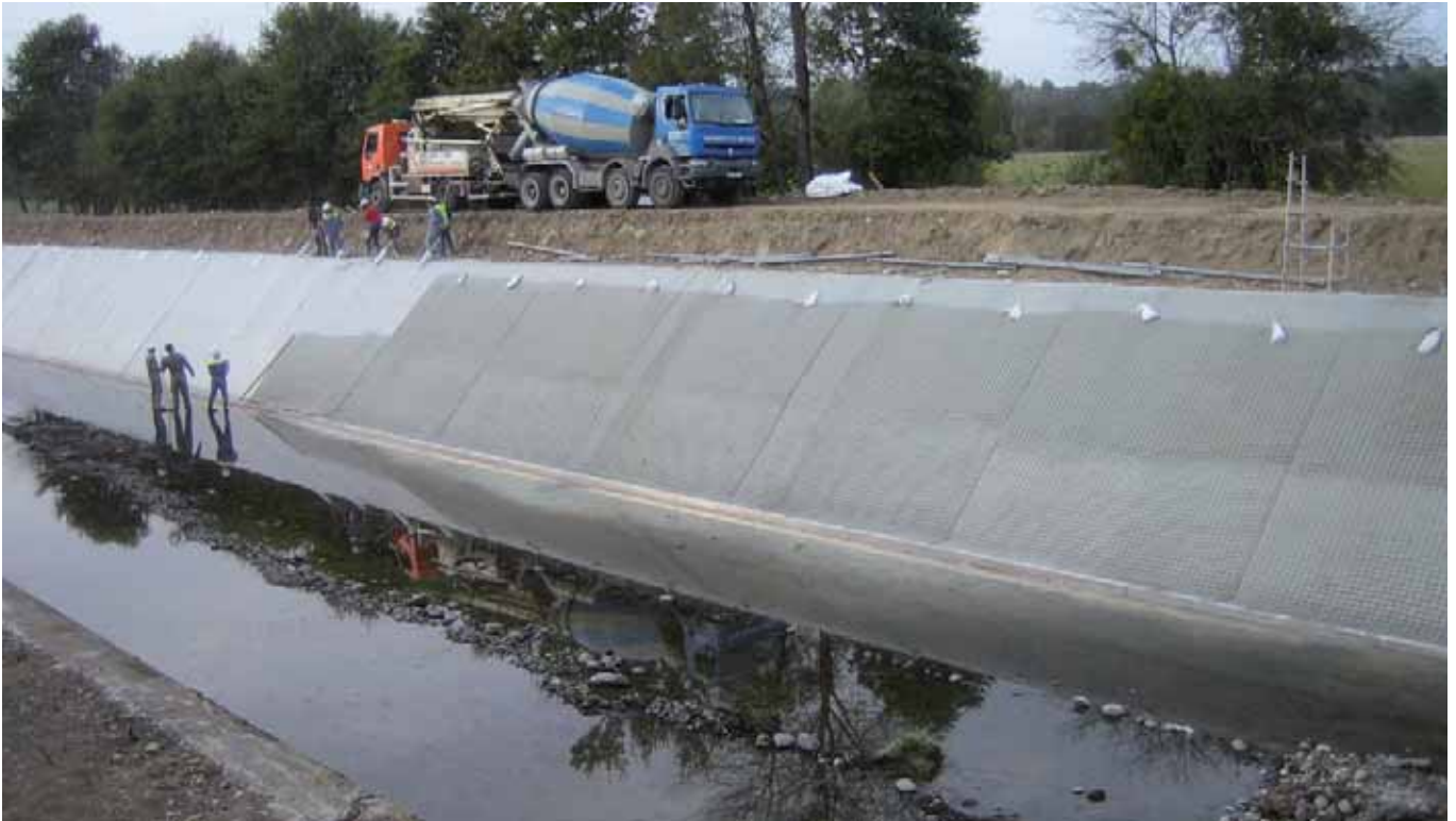
Progressive filling process of Incomat ®
