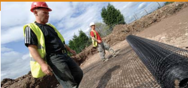
Installation of TriAx, Stoke
